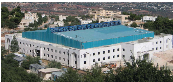
The SESAME building.
