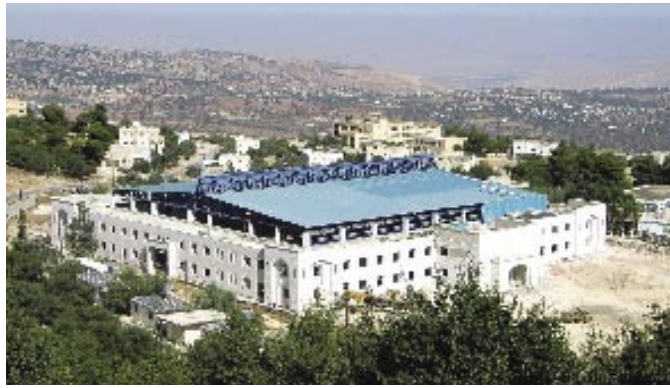
Hope for the future: SESAME under construction in Jordan.
