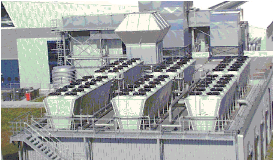
Figure 13.20: A picture of the 6 cooling towers used for the ANKA cooling plant.
