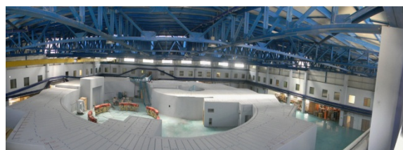
Figure1: SESAME Radiation shielding wall.
