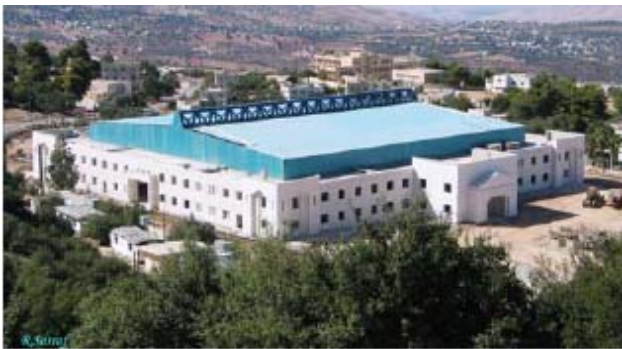
Figure 1: A panoramic view of SESAME building during construction (Nov. 2006).
