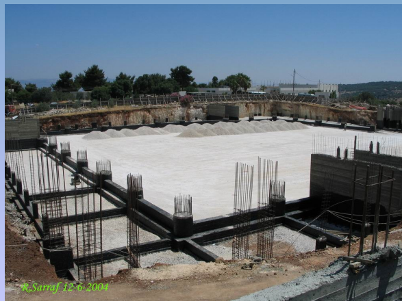
Progress Construction on Site
