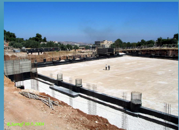
Progress Construction on Site
