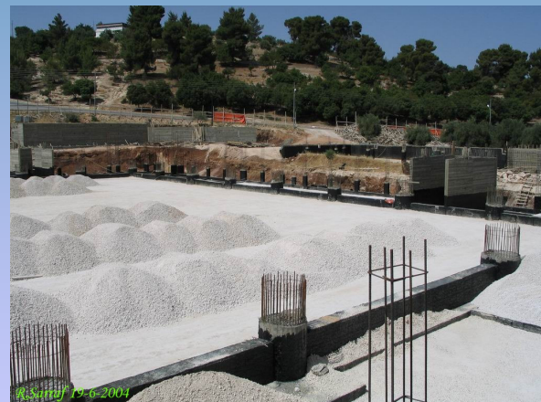
Progress Construction on Site
