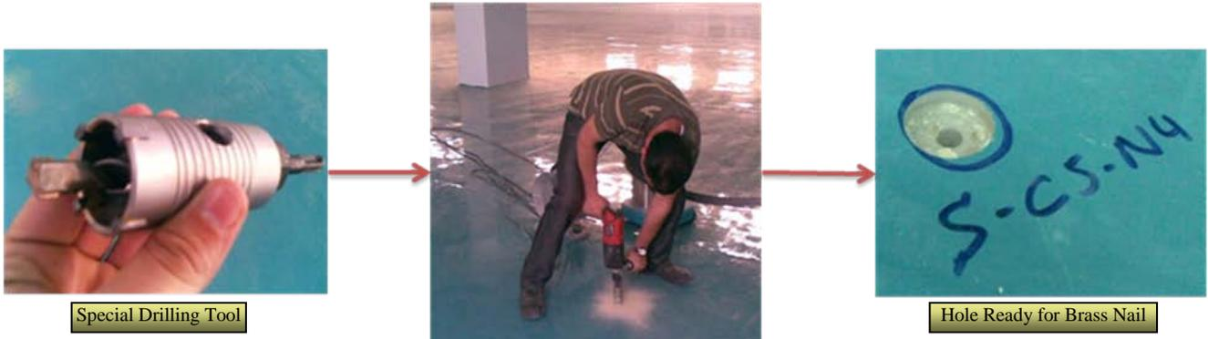
The nails sealing has been realized by means of the epoxy resin HILTI RE100.
