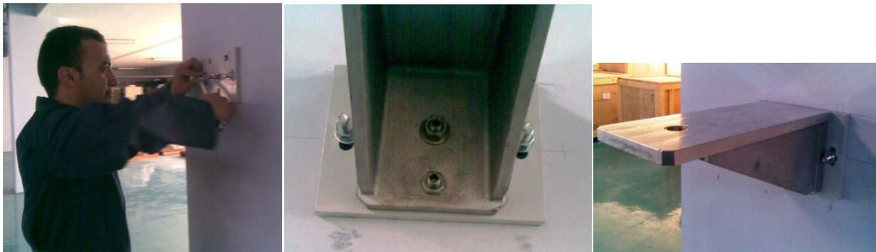
**Figure 8: the Installation of the Wall Bracket**
