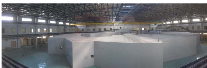
A view of the SESAME hall with completed shielding structure. The beamline apertures are clearly visible.
