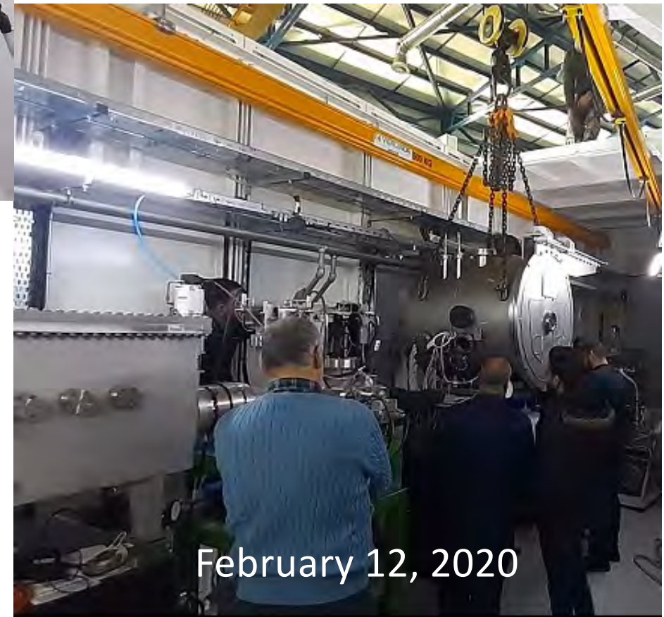
Installing the DCM Chamber
