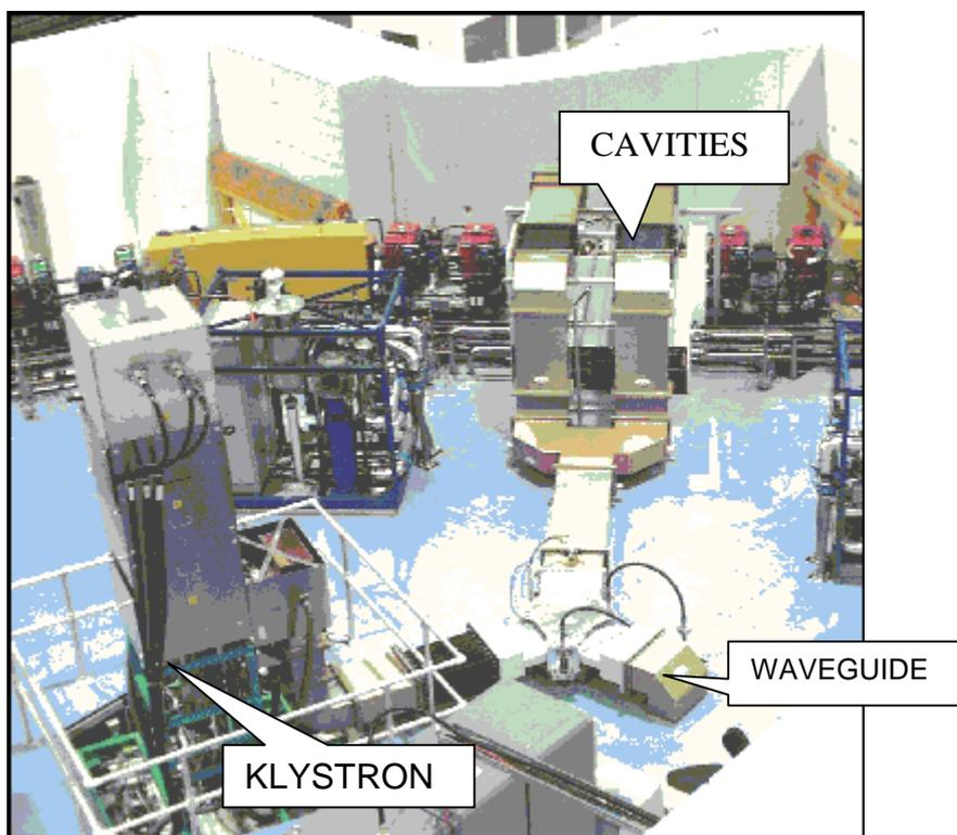
Figure 8.1: RF system of the ANKA storage ring. 250 kW microwave power is produced in the klystron. The power passes a circulator, which protects the klystron from the reflected power, split into two arms by a Magic T and coupled into two cavities.
